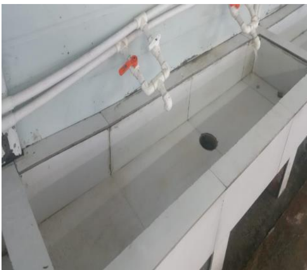
Current condition of hand wash facility
