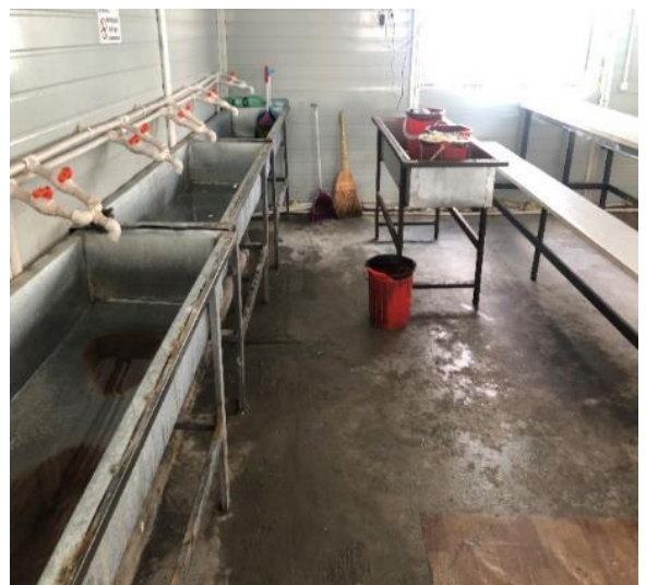
Previous hand wash facilities
