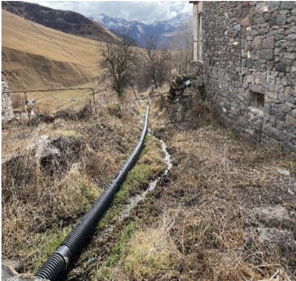
Pipe for temproyary septic system
